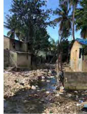
Damage from Hurricane Matthew, Dominican Republic
