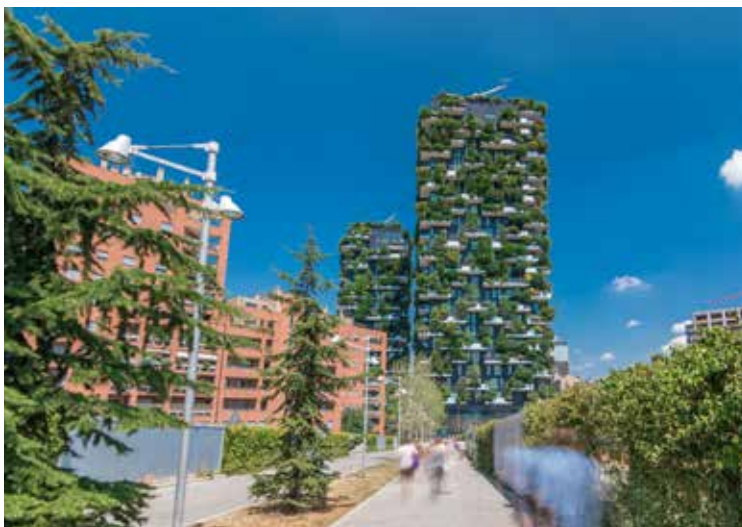
Two residential towers in the district of Porta Nuova, Milan, host hundreds of trees and plants in the balconies, Milan, Italy © Shutterstock
