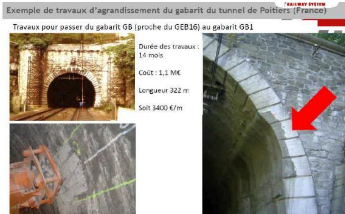
Figure 11: Tunnel vault works
