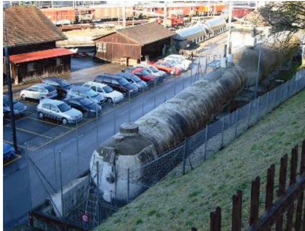
Figure 12. Switzerland liquified petroleum gas tank
